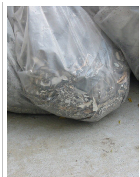
FIGURE 10.4 Paint chips should be double-bagged and seams sealed.
