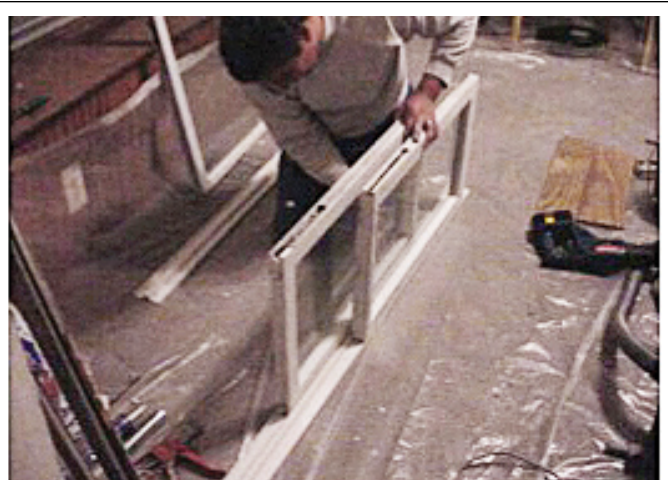
FIGURE 12.3 Replacement window system.
