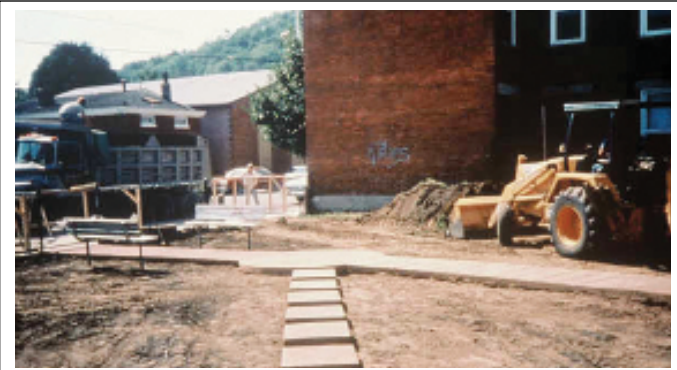
FIGURE 12.22 Replacing resident pathway after soil removal.
