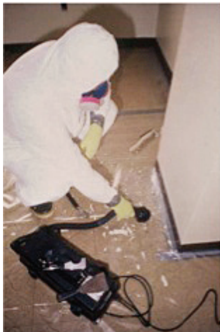
FIGURE 14.8 Vacuuming the floor containment.
