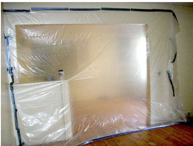
FIGURE 8.1 Prohibiting resident entry into work area by use of containment barrier.
