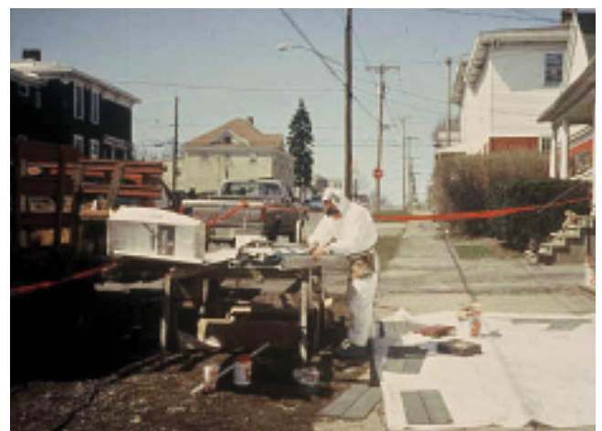
FIGURE 12.7 Certified workers are needed to replace siding when the project's intent is lead abatement.
