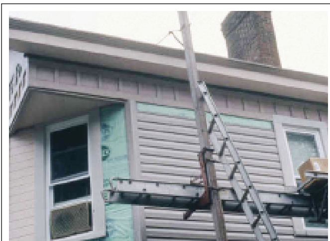
FIGURE 12.6 Installation of replacement siding.
